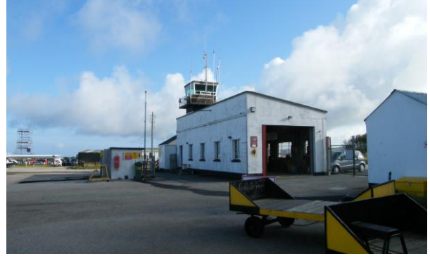
Land's End Airport will soon undergo major refurbishment including a new control tower.
